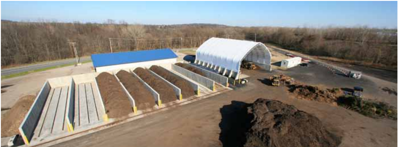
A birds-eye view of the newly renovated Amboy Compost Site. The Facility is the largest food scrap composting operation in New York State. It utilizes innovative, low maintenance “aerated static pile” technology which pumps air into the food and yard waste piles, eliminating the need to manually turn the piles. Learn more about the facility at OCRRA.org .
