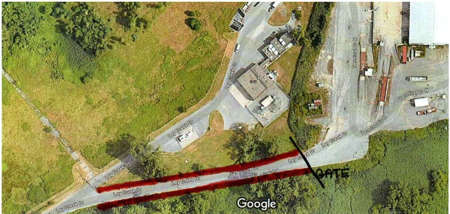
Ley Creek Transfer Station 5158 Ley Creek Dr. Liverpool, NY 13088
